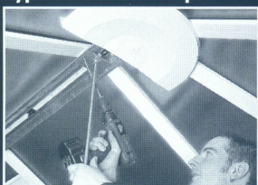
Fit the centre drop rod to the ridge body. The drop rod should be in-line with the brackets on the bars
