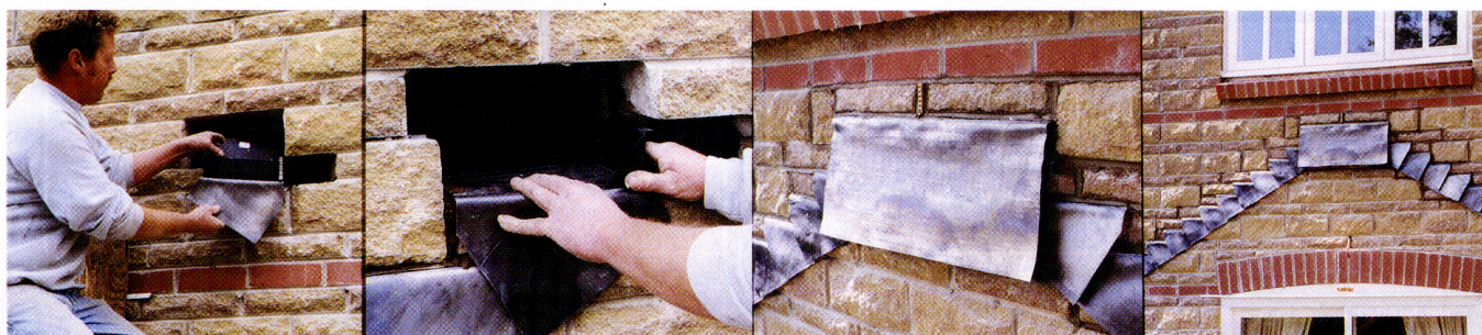
BELOW : A typical installation sequence.
