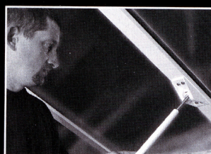
Screw the horizontal threaded bars into the brackets
